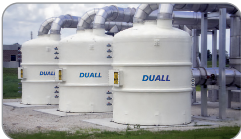
Activated Carbon Tower
