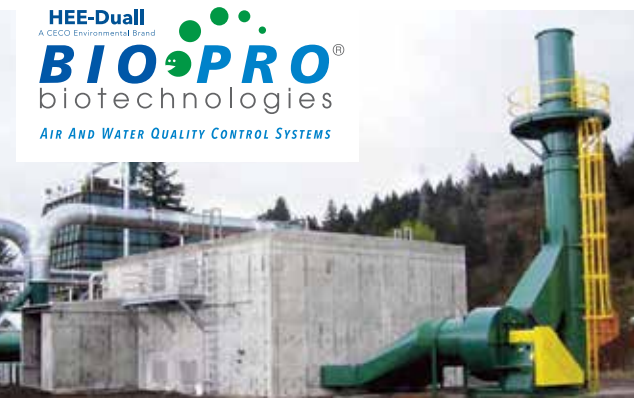
Biofilter Removing Hazardous Air Pollutants (HAPs)
