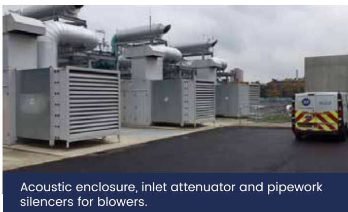
Ventilated enclosures and inlet attenuation for aeration plants.
