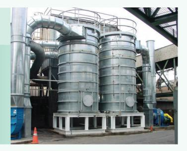
CECO Filters offers numerous styles of mist collectors based on state-of-the-art Fiber Bed Technology to capture and collect liquid mists, in particular sub-micron aerosol particles that cause exhaust stack opacity and blue haze. With our wide array of products and know-how we have the ability to provide the most economical and cost effective clean air solutions for your emissions problem.
