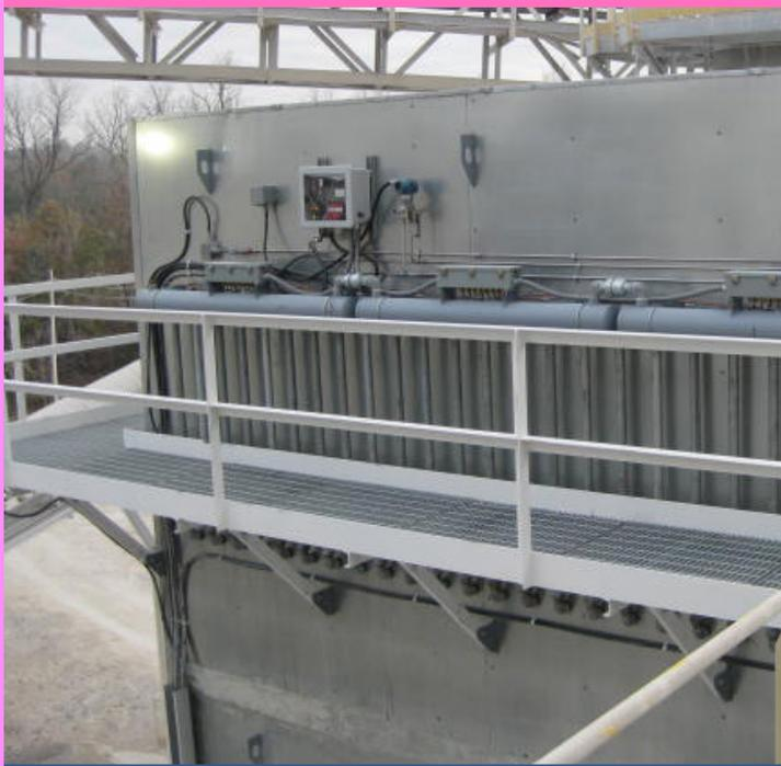
In addition, Mississippi Lime asked that the platform be 9" wider than Flex-Kleen standard and a wrap around the back of the walk-in plenum to mate to an existing ladder.
