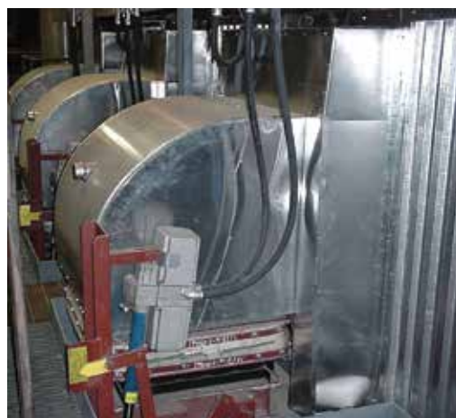
CCA's Overfire Air Ports
