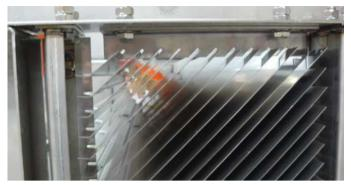
Depending upon the concentration of suspended solids and waxes, the plate spacing and plate inclination can be varied to suit the particular process conditions. This design flexibility enables us to offer our clients a technically optimised solution for each individual application.
