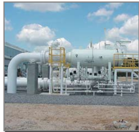
THIS PEERLESS FILTER-SEPARATOR IS INSTALLED AT A COMPRESSOR STATION IN NATURAL GAS TRANSMISSION SERVICE. THIS PEERLESS UNIT IS DESIGNED WITH A COST-EFFECTIVE FULL-DIAMETER CLOSURE.
