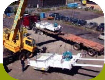
**Flextor offers a complete line of heavy-duty guillotine dampers to meet your requirements.** We have installed dampers in ducting sizes as large as 25' high by 16' wide. Our zero-leakage designs have been hydro-tested as high as 3 PSI and hydro tested at 60 PSI for structural integrity.
