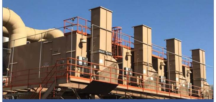
SECONDARY EMISSIONS CONTROL FOR LEAD AND METALLURGIAL FUMES
