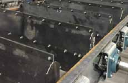
AIR HEATER ISOLATION LOUVER
