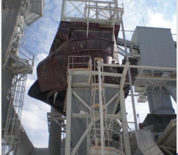
The original dust collector included 300 filters, featured panelized construction, and was fabricated in Austria and assembled on site with hopper heat tracing and insulation.
