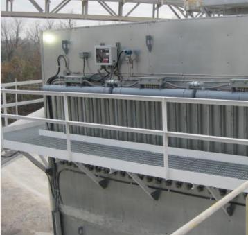
In addition, Mississippi Lime asked that the platform be 9" wider than Flex-Kleen standard and a wrap around the back of the walk-in plenum to mate to an existing ladder.
