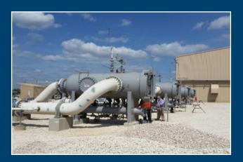
ULTRA filter-separators installed in parallel for final cleaning of natural gas before liquefaction.
