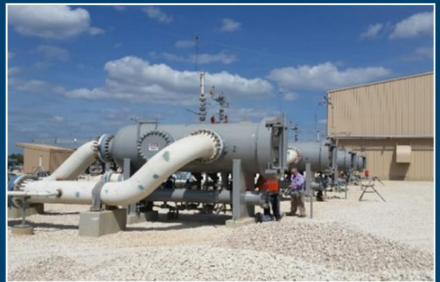
ULTRA filter-separators installed in parallel for final cleaning of natural gas before liquefaction.
